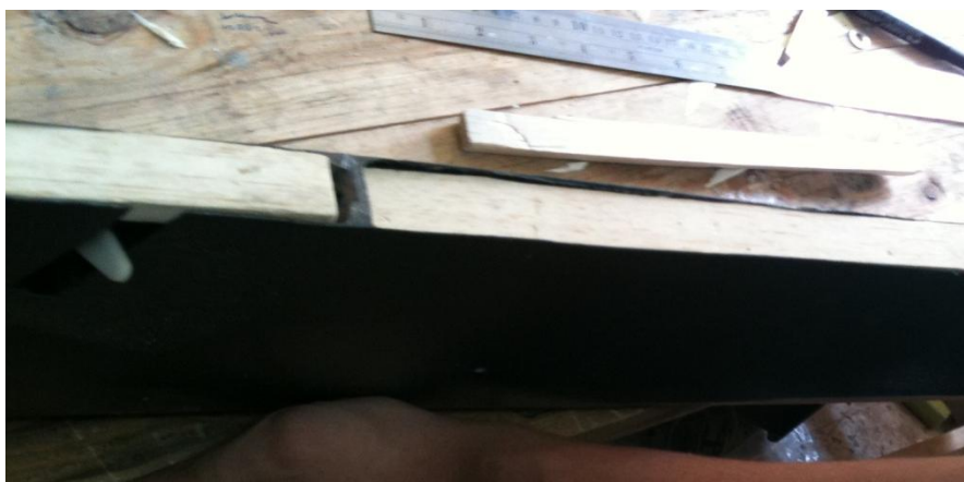
Figure 136: Filling empty edges
