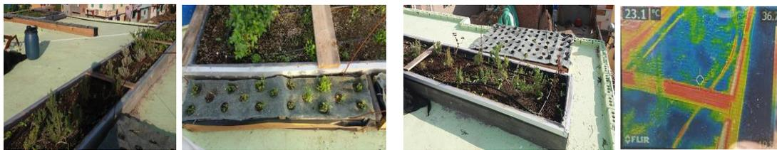
a) Green roof with herbs and vegetables      b) Thermal image after installing the green roof
