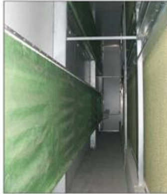
Tunnel inlet with roller curtain
