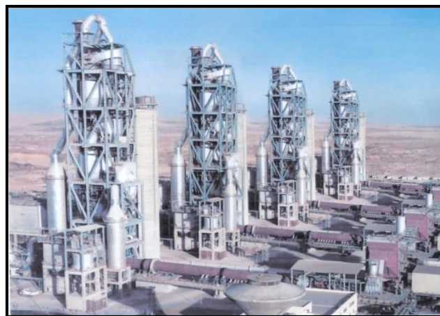
Fig 9.3 Typical view of a cement factory
