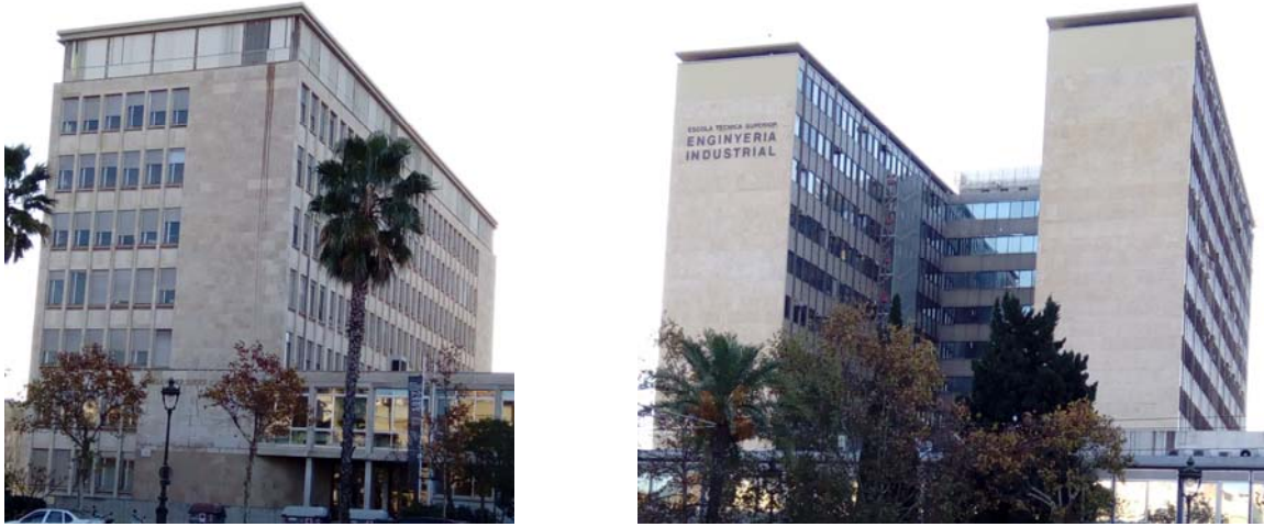
Figure 3. The Architectural Engineering School building (left) and Industrial Engineering School building (right).
