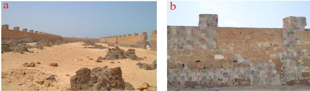
Fig. 14. (a) Collapse of Parts of the Building, (b) Erosion of Mortar Layers and the Building's Limestone
