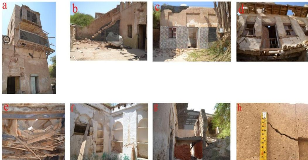
**Fig. 20. (a) Damage on the Facades of Abdullah Ibrahim Al-Rifai's House, (b-d) Spread of Structural and Architectural Problems, (e-g) Collapse of Parts of the Building's Roofs, 20h. Spread of Cracks**
