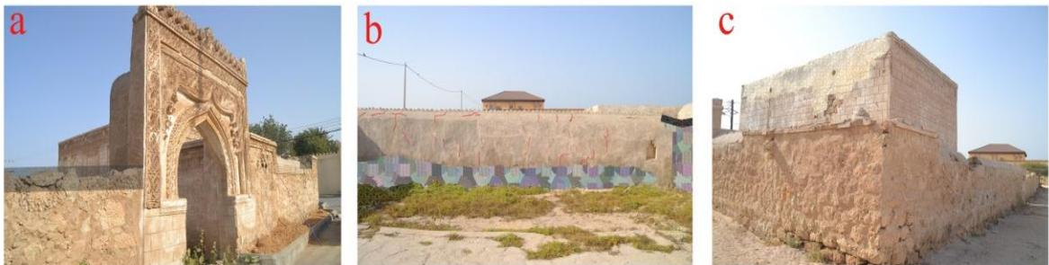
Fig. 18. Deterioration Phenomena in Hussein Al-Rifai's House: (a) where Parts of the Building Collapsed, (b) The Falling of Casing Layers and Mortars, (c) Inappropriate Restoration Work
