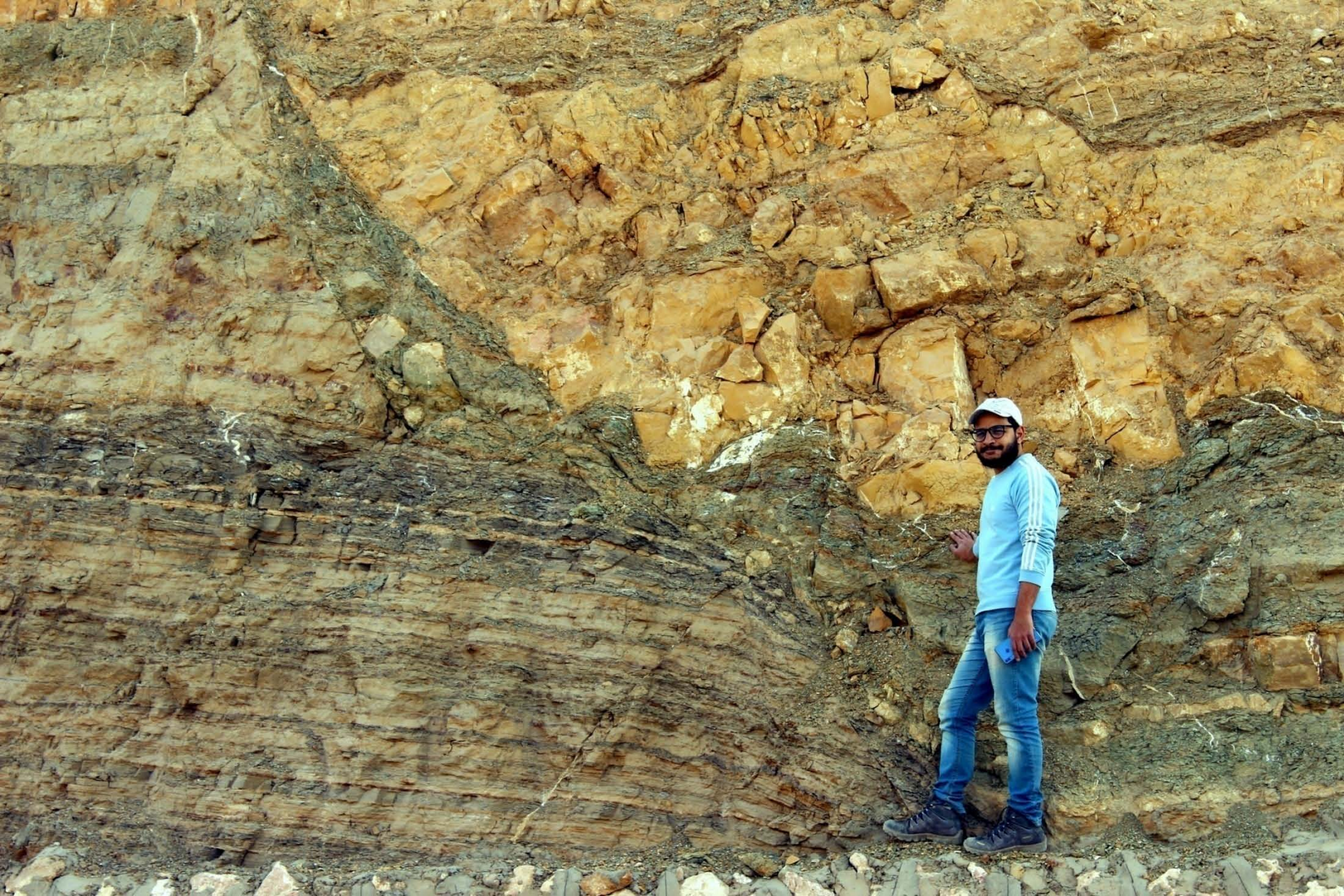
Normal Fault in sandstone and shale layers causing dragging of beds and shale smearing
