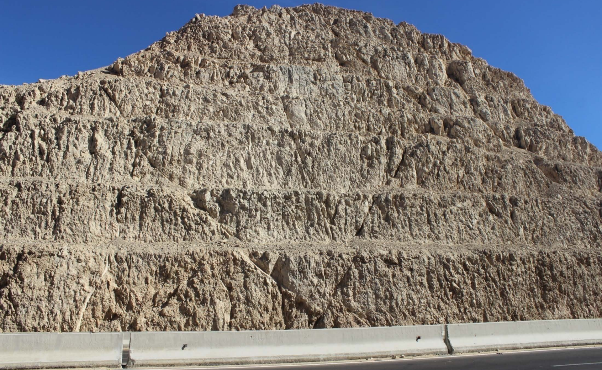
Two conjugate sets of shear joints in limestone beds
