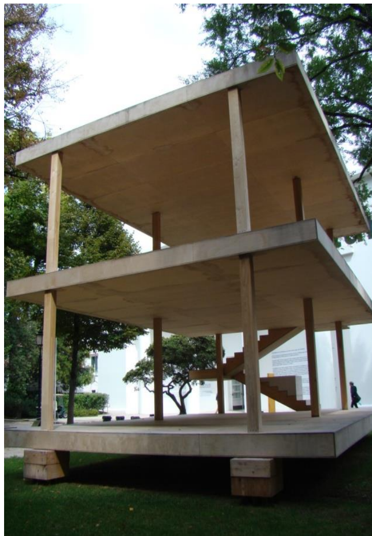
1:1 model replicates Le Corbusier's Maison Dom-ino, by Rem Koolhaas, Entrance to "Elements of Architecture", Author, 2014
