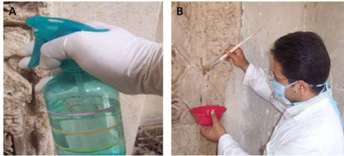
Fig. 11. The application of the solutions: a – fungicide, b - Eucosil consolidant
