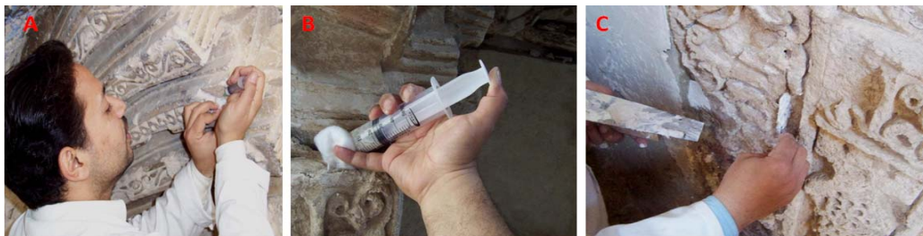
Fig. 8. Images during treatment: a - adhesion of detached pieces of stucco decorations, b - the injection of stucco decorations, c - the mechanical strengthening of stucco decorations by mortar.
