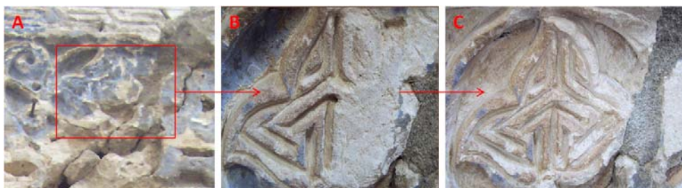
Fig. 6. Stages of revealing of the disappeared motives by mechanical cleaning
